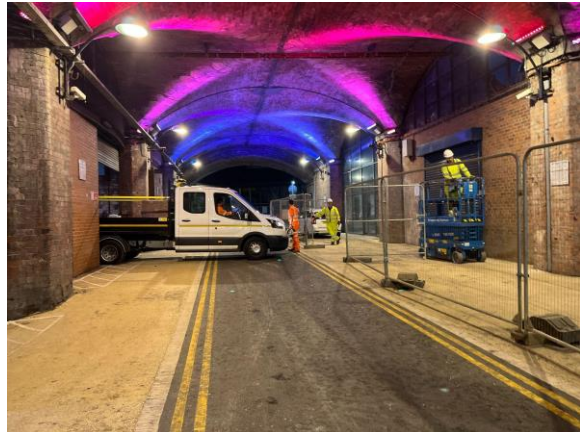
Dark Neville Street Arch Entrance
