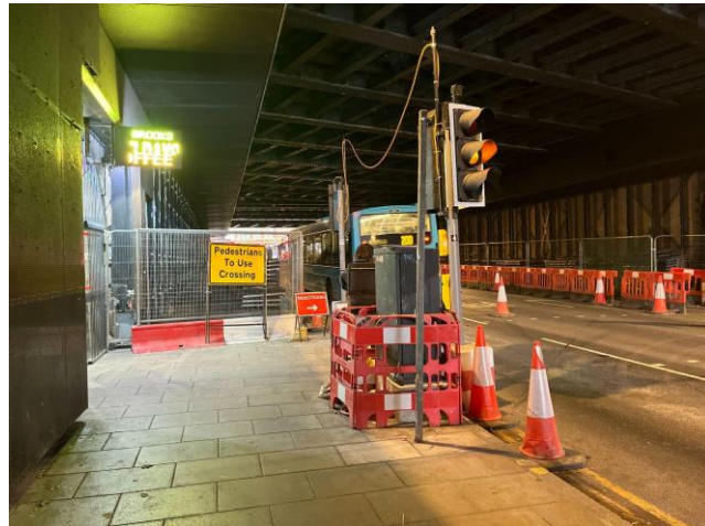
Road works outside the Dark Neville Street
